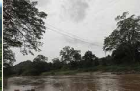
Photo 14: Orang-utan rope bridge constructed along Segama River to provide connectivity for orang-utan from Bukit Piton Forest Reserve to USM
