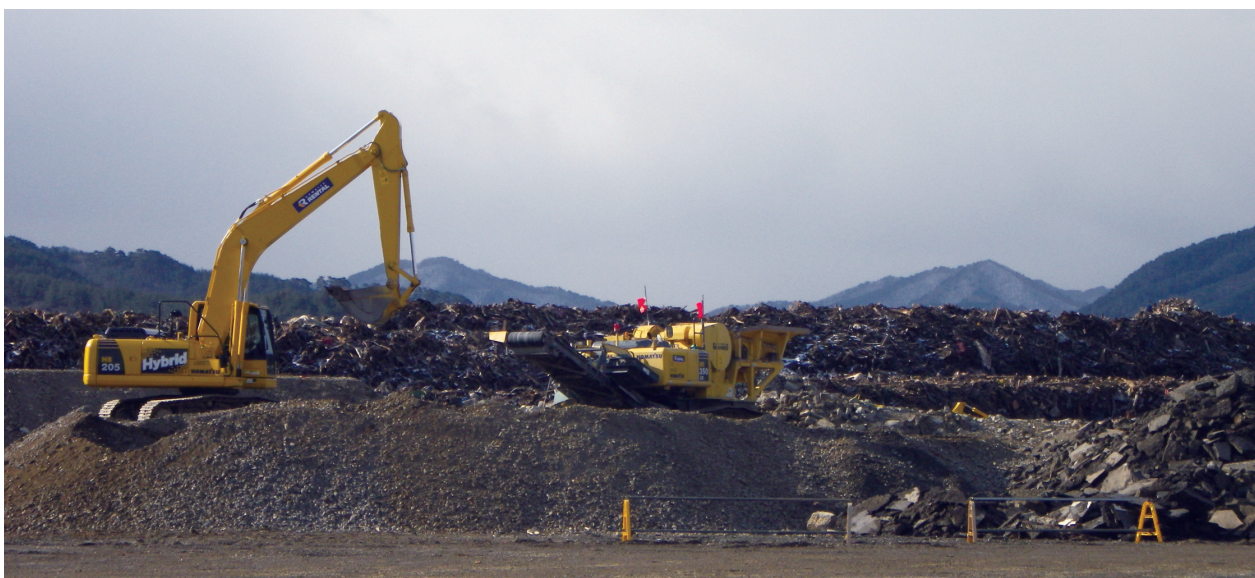
Restoration work in progress (Minamisanriku Town)
