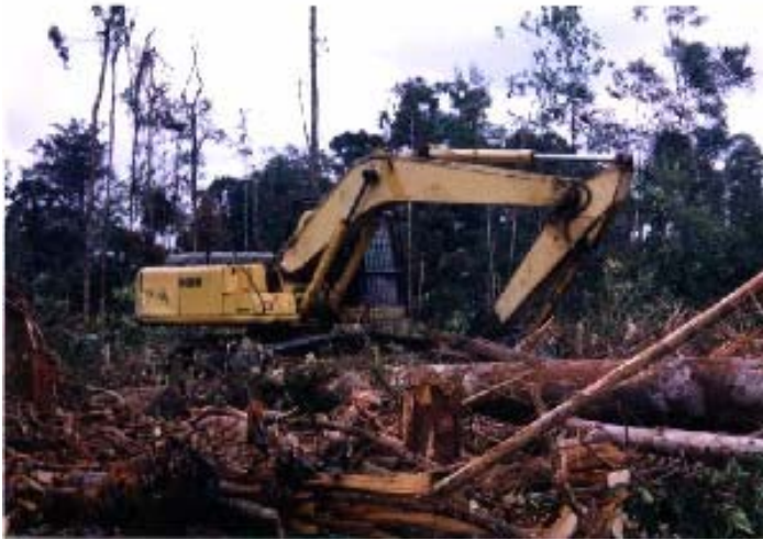
Figure 7. Excavator used in the professionally executed operations of Group 'W' (Photo taken on 1 June 2003)
